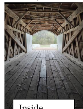
Inside Roseman Bridge
